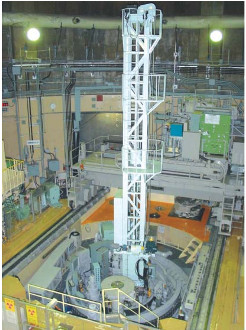
The Joyo sodium-cooled fast reactor, in Japan. Development of the GFR reactor line calls for irradiations in experimental fast reactors, such as Joyo, and Phénix, to test innovative fuels and materials.
